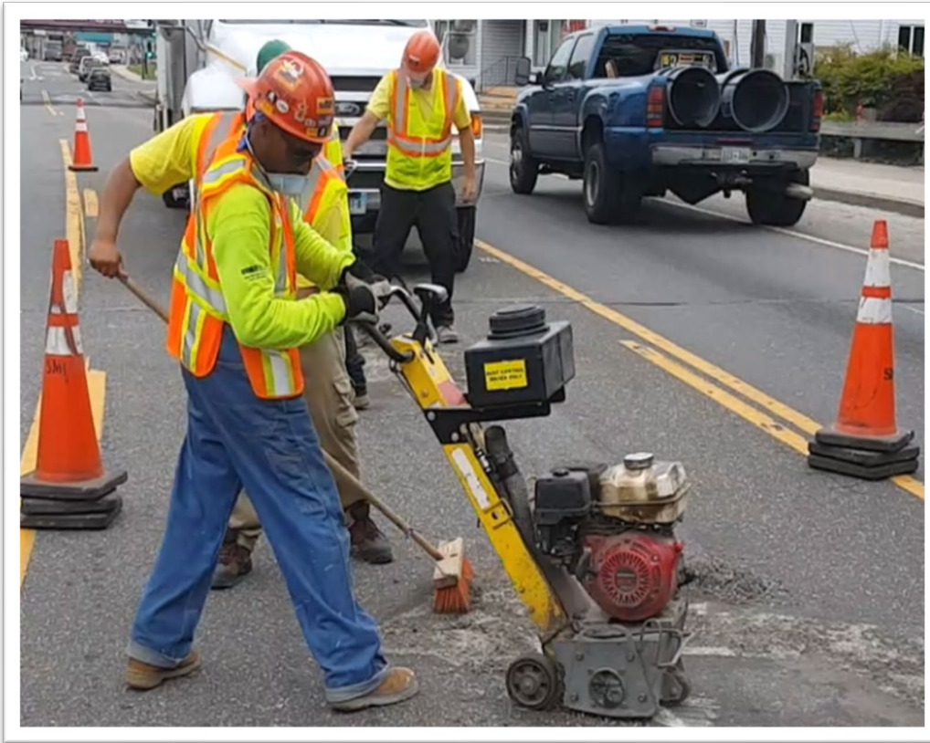
Figure 1: Hand grinding a left-turn arrow (tape), to replace with epoxy, using the Von Arx VA25s scarifier.
