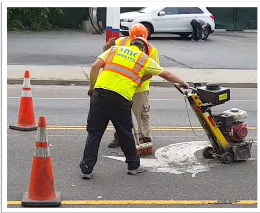
Figure 3: Allowing the sweeper to keep pace so debris doesn't gather under the grinder.
